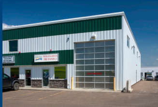
FIRE STATION 23 37 Burnt Basin Street Red Deer County, AB
